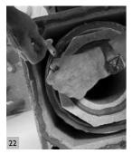
4x steel spacers push fitted around inner flue block every 1m of chimney.
