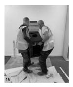
Now slide the appliance into position and adjust and fix using the 3 screws at the bottom.
