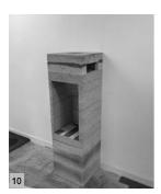
Apply glue before fixing the top plate in position.
