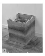
Apply glue to the module outer edge, with the exception of the gap for the first ventilation grill.
