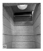
Push the long end of the air outlet up through the slit in the top plate on the frame, and put 2 layers of fibre tape around the protruding air outlet before sliding them down to seal the gap around the outlet.
