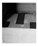
Glue the 3 metal plates onto the base plate within the opening for the insert so they lie under the 3 adjustable feet (bolts) in the bottom of the appliance.
