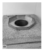
The Octagonal stainless steel adaptor slides down inside the stainless steel pipe shown previously. The bottom of the Octagonal adaptor lies flush onto the Pumice top plate.
