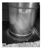
The steel pipe is sealed into the stove using fire cement.
