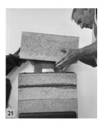
The first outer chimney block is glued into place, making sure it's square and level.
