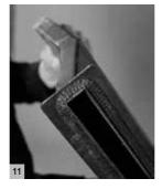
Fasten fibre tape once around the underside of the flange of the air outlet.
