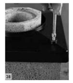
Fix capping using the bolts provided.
