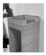
Apply glue to each block edge, with the exception of the gap for the 2nd ventilation grill
